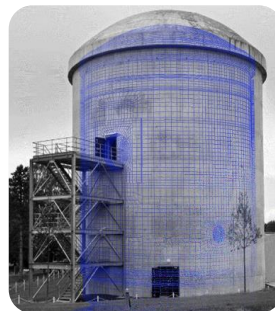
VERCORS mock up and its digital twin
